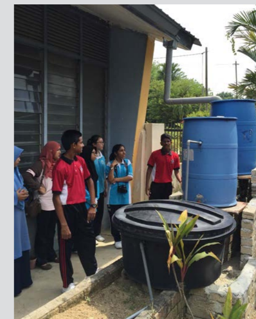
Setting up a water harvesting system in a school.
